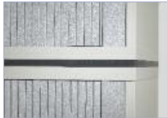
Gestaltungselement Schattenfuge Shadow gap as a design element
